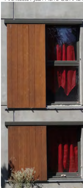
Panneaux bois coulissants (Magny-en-Vexin)
